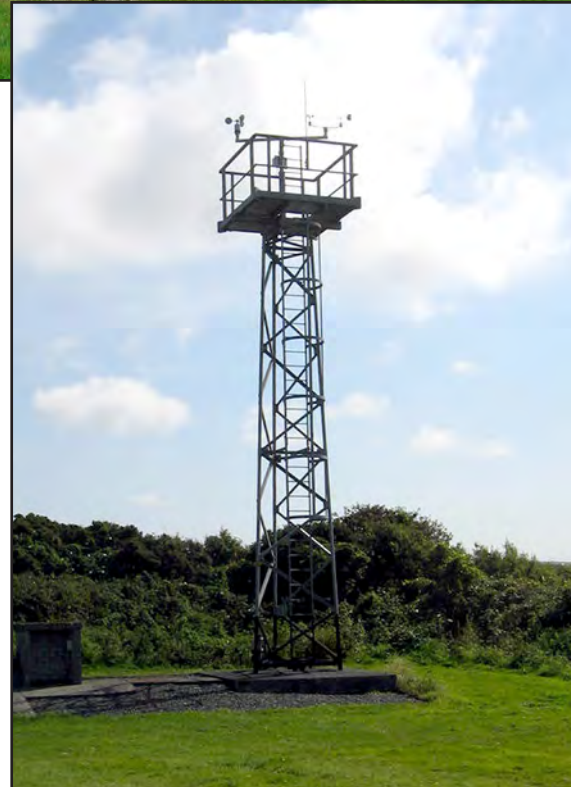
Figure 2. Camborne wind tower.
