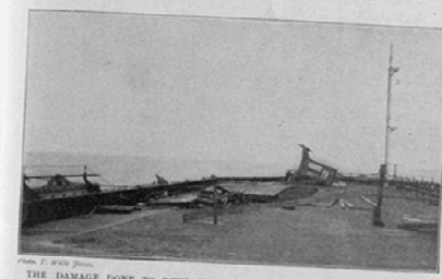
THE DAMAGE DONE TO RHYL PIER, SHOWING THE OVERTURNED KIOSK.
