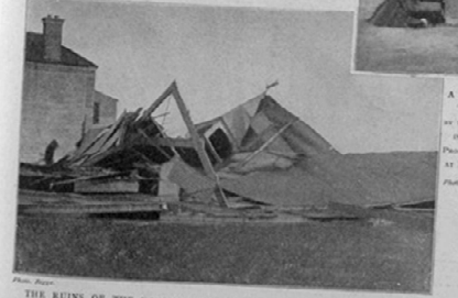
THE RUINS OF THE ROMAN CATHOLIC IRON CHURCH AT GREYSTONES, BLOWN DOWN ON FEBRUARY 26.
