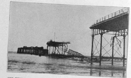
THE WEST END OF PIER, MORECAMBE, AFTER THE STORM OF FEBRUARY 27.
