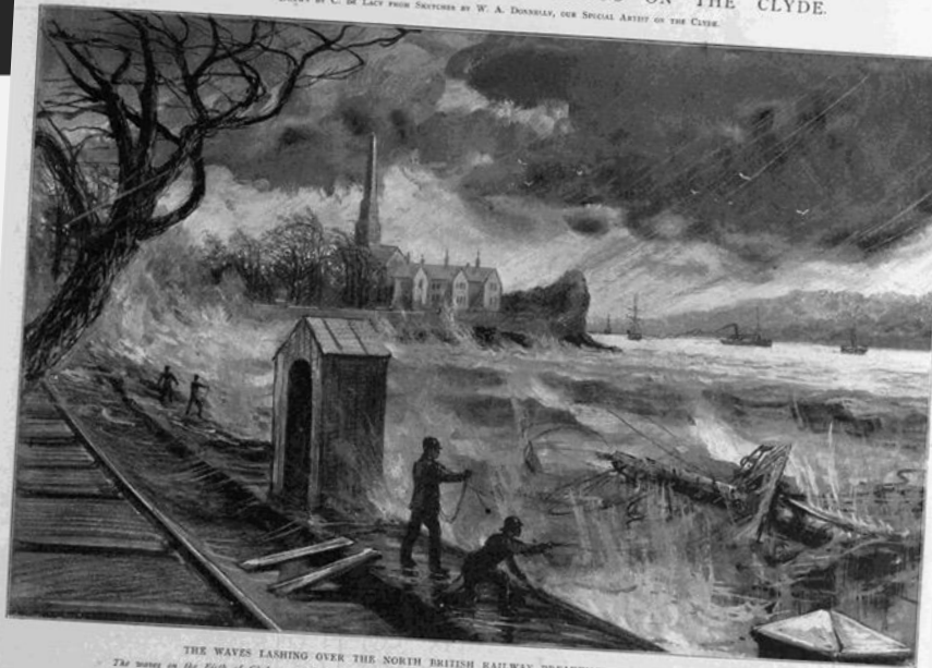
THE WAVES LASHING OVER THE NORTH BRITISH RAILWAY BREAKWATER AT DUNGLASS CASTLE. The waves on the Firth of Clyde were of unprecedented height. In noon on February 20 the wind blew a hurricane, and all craft ran for shelter.
