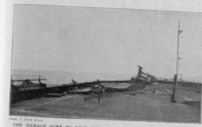
THE DAMAGE DONE TO KILLY PIER, SHOWING THE OVERTURNED KIOSK.
