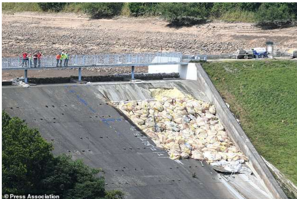
Fig G.2: Work to shore up the dam spillway
