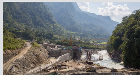
Construction of the Upper Marsyangdi Hydroelectric Station.
